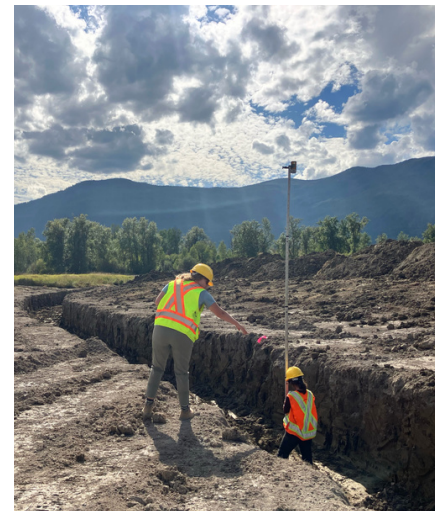
Workers using a laser level to measure the depth of the newly constructed channel at the 2023 Yaqaan Nukiy restoration site.
