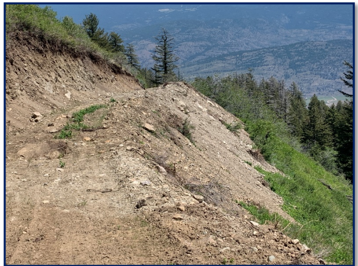
Figure 6. Government caused damage to the environment when it constructed this unauthorized trail for a water diversion.
